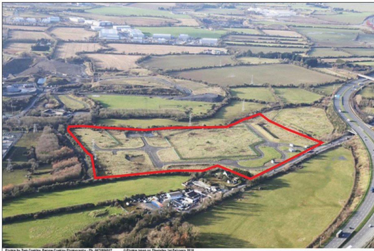
Figure 1-2 Existing Aerial Image of the RBSF site from the East
