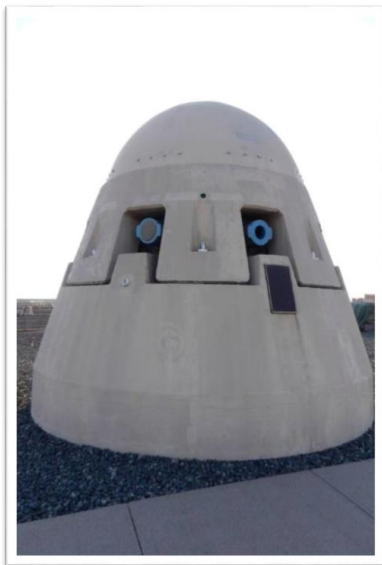
Diagram 5-5: Precast Concrete Protection to Diffuser Valve
