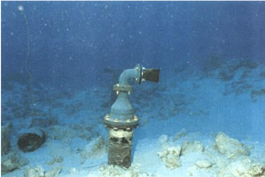
Diagram 4-2: Typical Diffuser Valve at Seabed Level (courtesy of Tideflex (2018))
