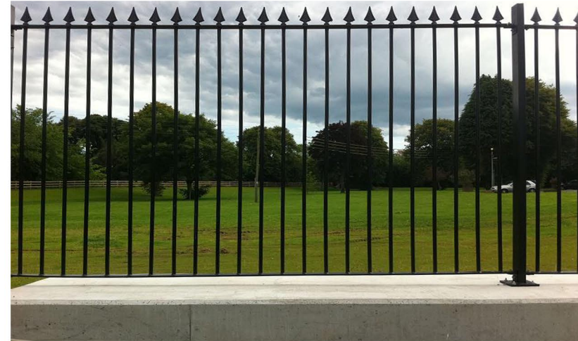
Fig.1 - Ornamental system railing security fence. Circa 2.5m high
