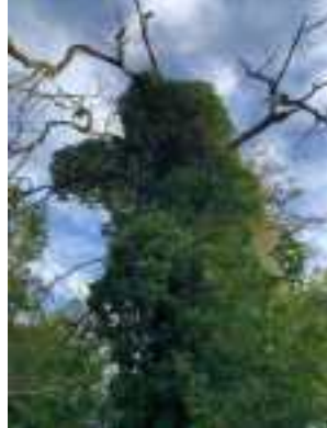
Partially detached ivy with stem diameter in excess of 50mm/Low
