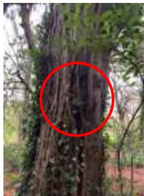
Knothole from shed branches/moderate
