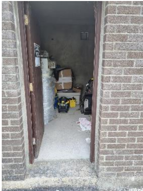
Figure 2: Disused Fluorine Room
