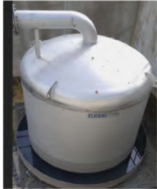
Figure 3: Lifford WwTP CWF Storm Flush Image 2
