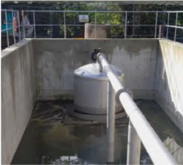
Figure 2: Lifford WwTP CWF Storm Flush Image 1
