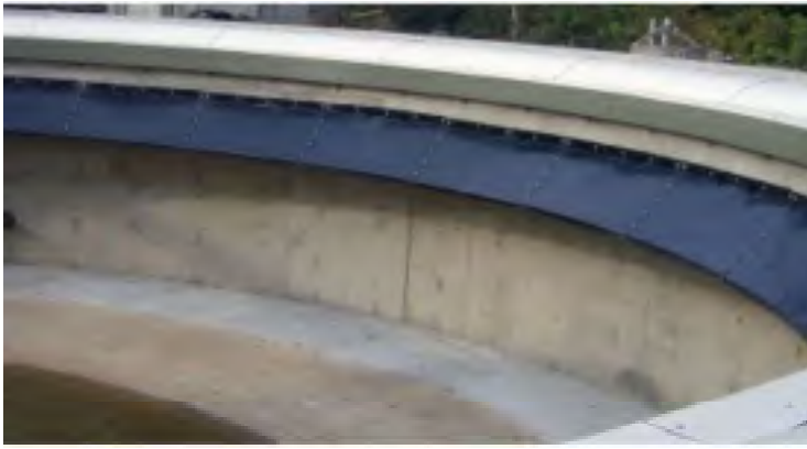
Figure 15: Stamford Baffle
