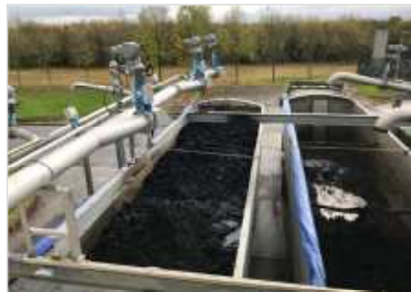
Figure 20: Bunlicky WwTP Dewatered Sludge Storage
