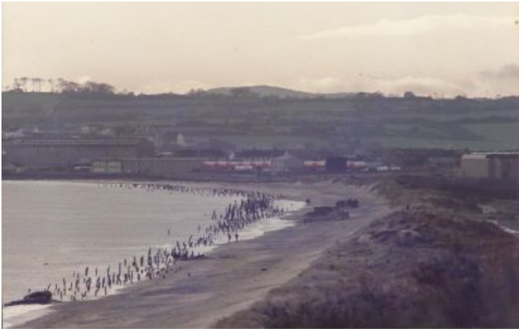
Figure 16: Beach and dune system with vertical piles remaining from previous defence structure. Date unknown.
