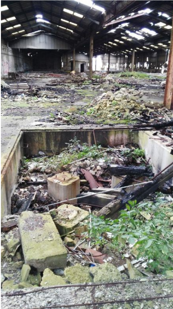
Photograph 13: Pit inside factory building, facing south.
