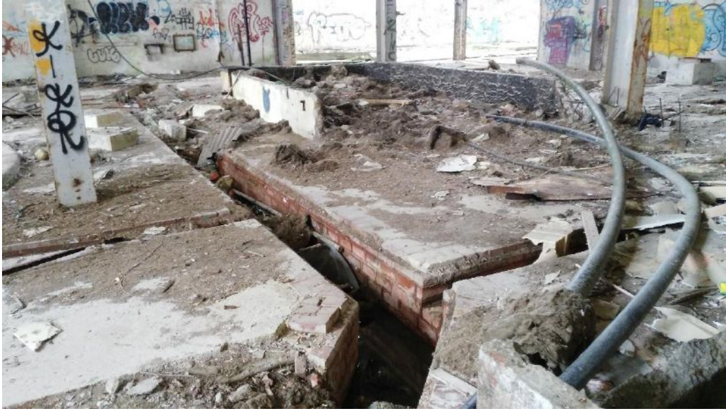
Photograph 14: Trenches inside factory building.
