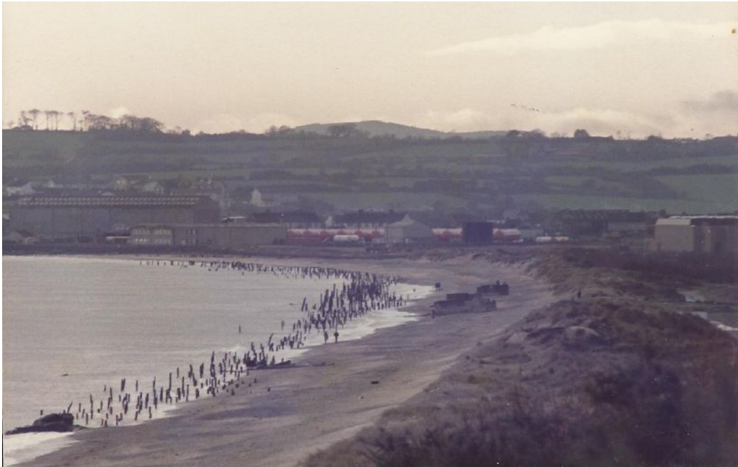
Photograph 10: View facing south showing coastal erosion protection on beach with the Wallboard Factory in the background, unknown date.
