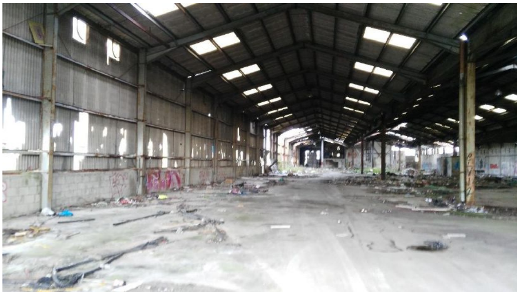
Photograph 12: Inside factory building, facing north.
