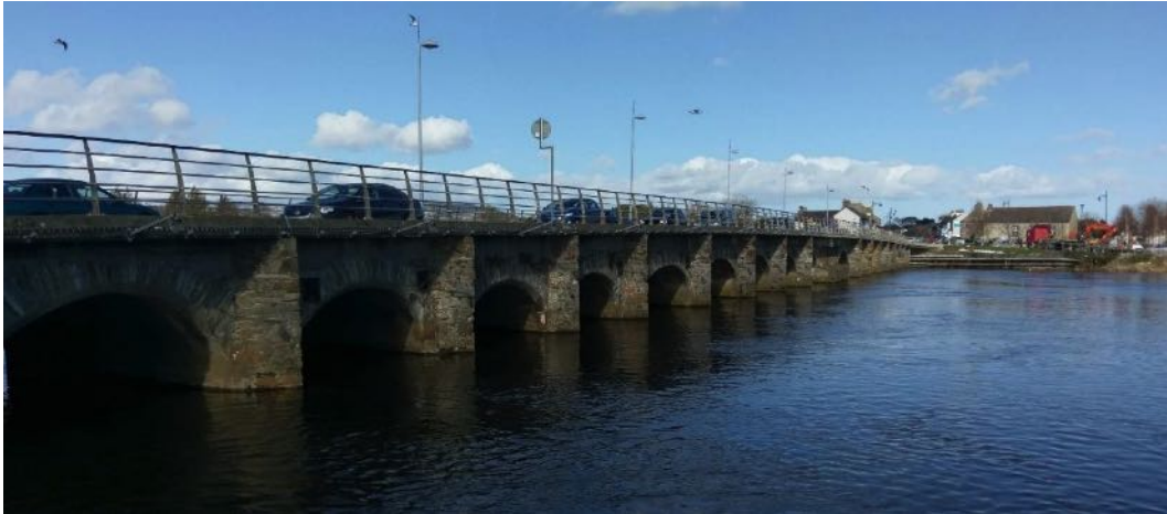
Figure 13.7: Arklow Bridge seen from South Quay
