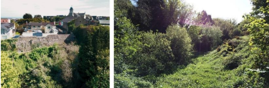
Figure 13.3: The Alps escarpment, from elevated and ground level, looking south towards the rear of the buildings on Upper Main Street
