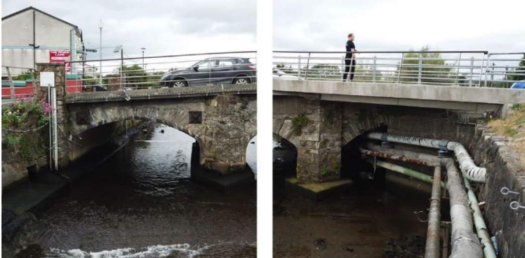
Figure 13.8: Downstream view of the first (southern) and nineteenth (northern) arch of the Arklow Bridge
