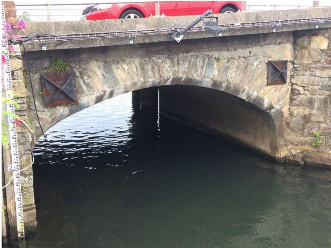
Figure 12.10: Southernmost arch of Arklow Bridge (RPS A26), facing northwest
