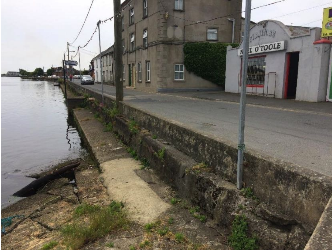
Figure 12.13: South Quay wall, facing south-southeast
