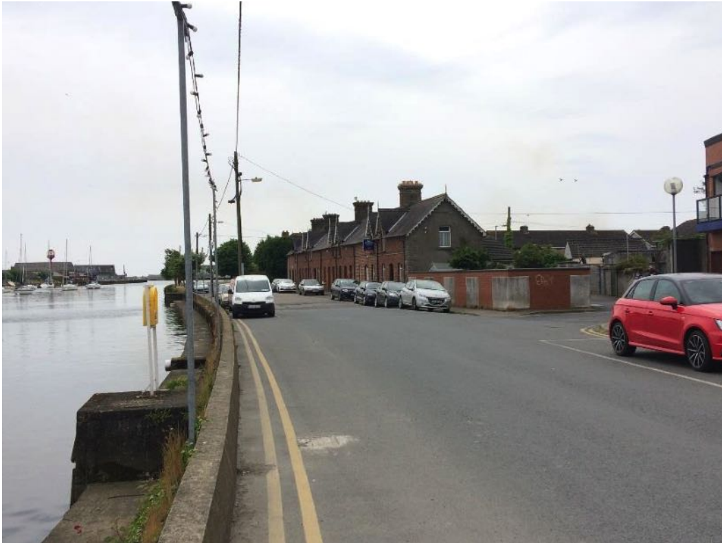
Figure 12.12: South Quay, facing southeast
