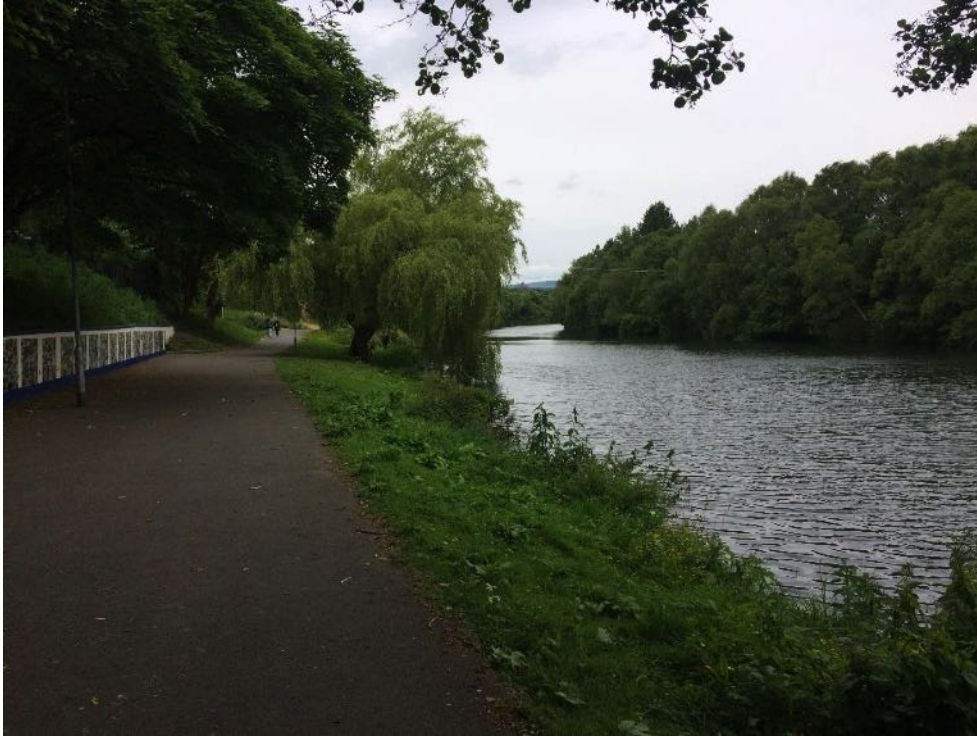
Figure 12.7: Route of proposed interceptor sewer adjacent to the Avoca River, facing west (upstream)
