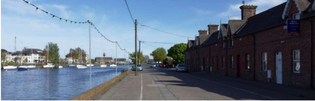
Figure 13.9: South Quay looking downstream, with residential buildings directly facing the quayside
