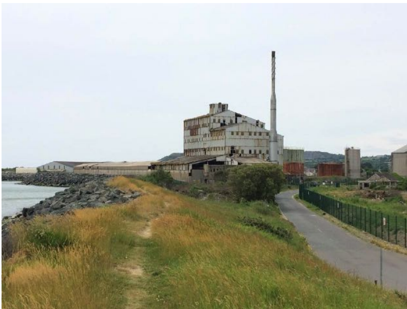
Figure 12.18: WwTP site with coastal rock armour, facing south
