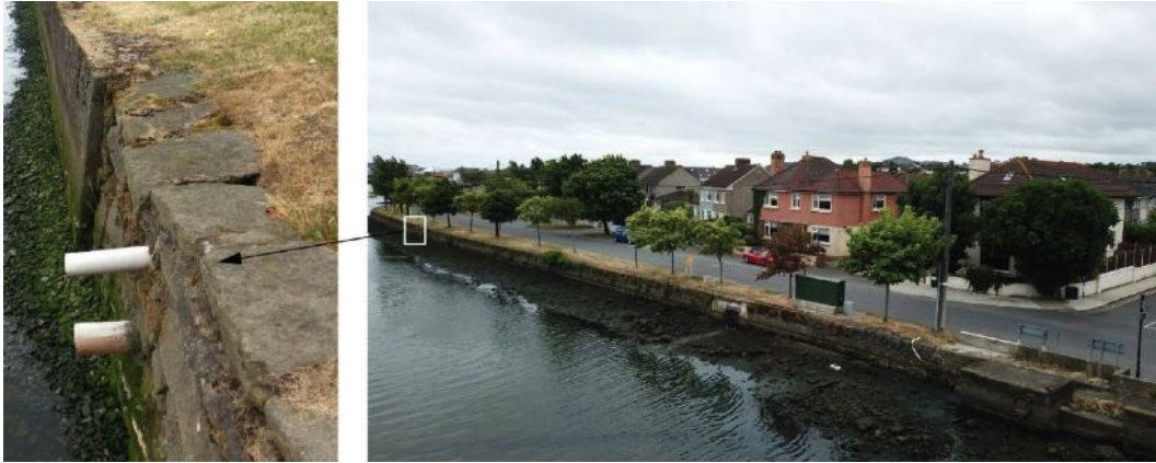
Figure 13.14: Section of quay wall where rubble stone remains visible and stone flags form top of wall
