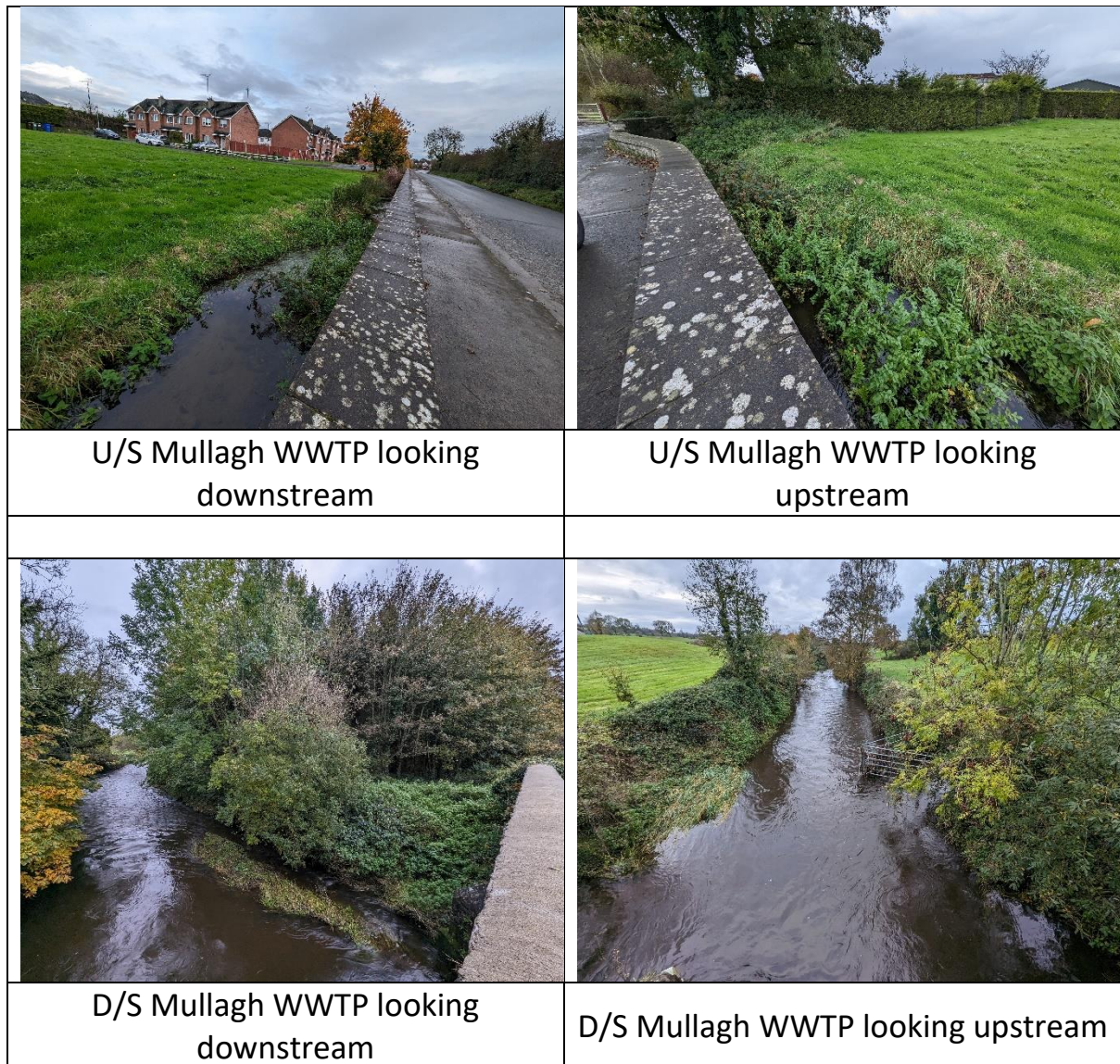
Figure 2. Upstream (U/S) and downstream (D/S) of Mullagh WWTP.
