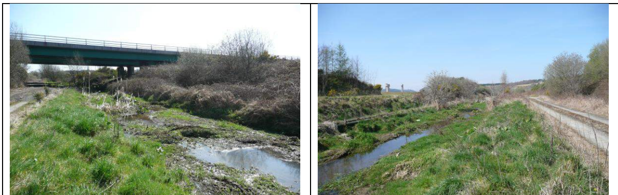
Plate 6. Canal and adjoining access track at Shelton Abbey. Left, looking east, the Sheepswalk stream is culverted under the track and into the canal; Right, looking west.
