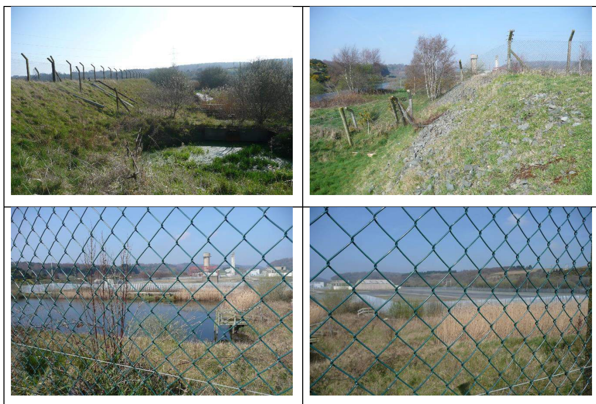
Plate 3. Shelton Abbey, lands south of Plot A. Top left, Canal at north east corner of site showing sluices and aquatic vegetation; Top right, embankment at south east corner of site showing Avoca River and floodplain to left; Bottom left, Reservoir with fringing reedbed; Bottom right, smaller reservoir with reedbed; un-vegetated areas of site can be seen in the background.
